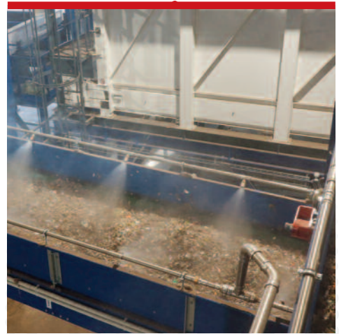
Sprinkler firefighting systems for separation hoppers
